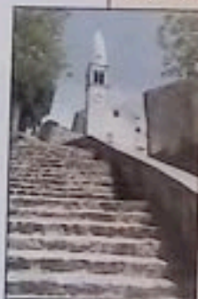
54. The late Gothic church of Štanjel built in the XV century and rebuilt in the XVII century housing Counts Cobenzls' tomb
